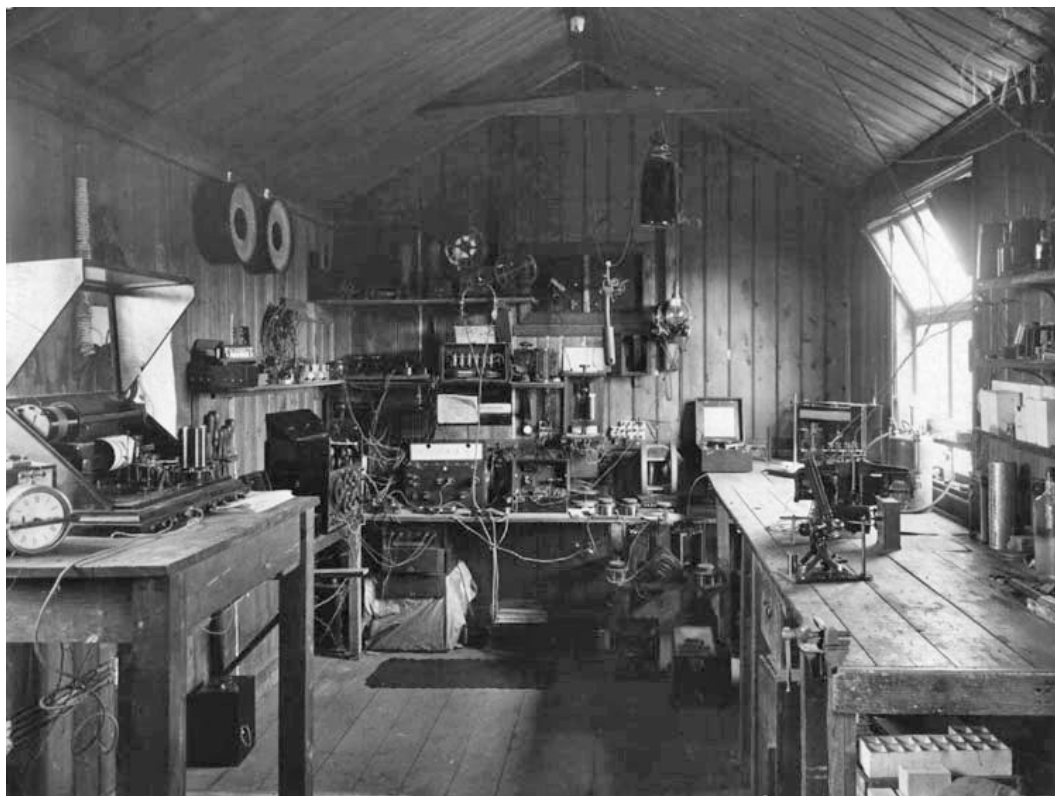
Fig. 18 The interior of the Meteorological Office Radio Station at Smallshot Bottom photographed in 1919. The lightning recorder is the large instrument on the table to the left. (Rutherford Appleton Laboratory)
