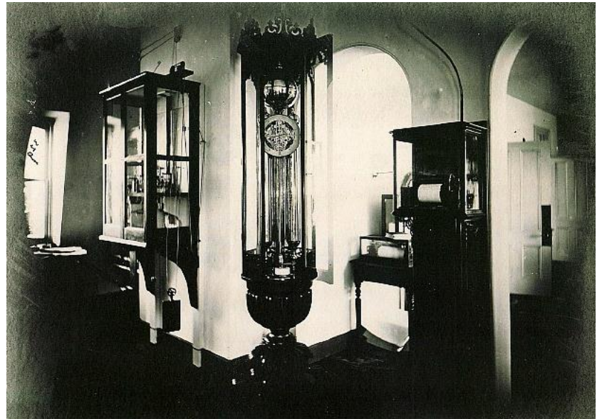
The inside of General Myer's Headquarters, showing, left to right: self-registering barograph designed and produced by Professor George Washington Hough at the Dudley Observatory in Albany, NY; Rochester Barograph, most likely produced at a shop in Downtown Rochester, New York; Gibbon Rain Gauge, named after David John Gibbon.
